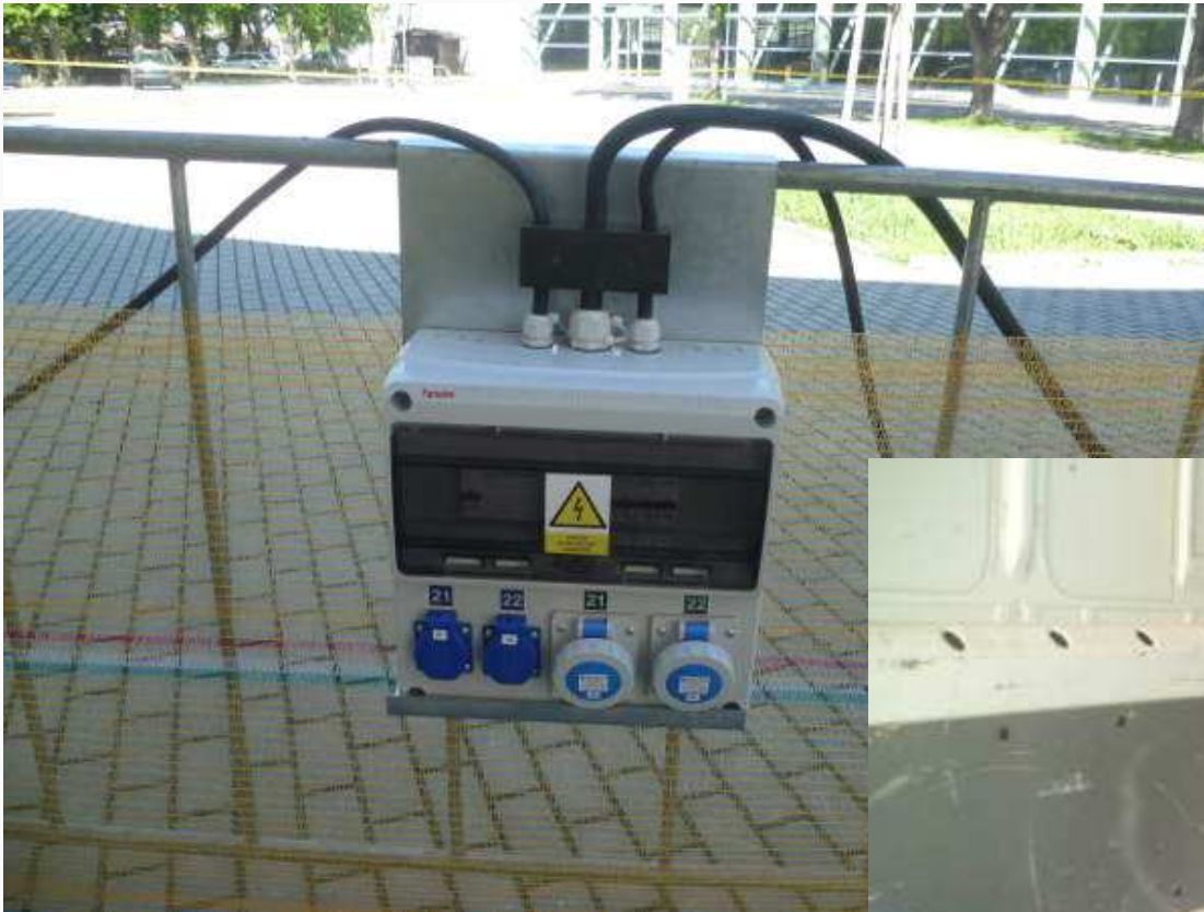
Electric panel with N. 2 single-phase IEC 309 16 A sockets and N.2 Shuko sockets
